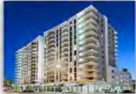
Grove Station / ZOI House
